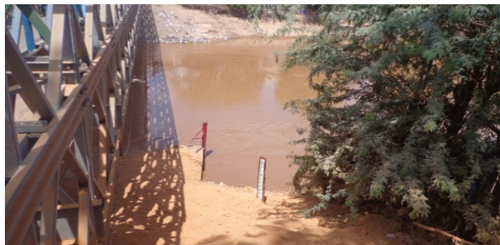
Figure 4.16: Jowhar staff gauging station
