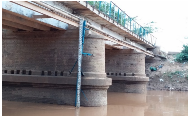
Figure 4.19: Jowhar staff gauging station
