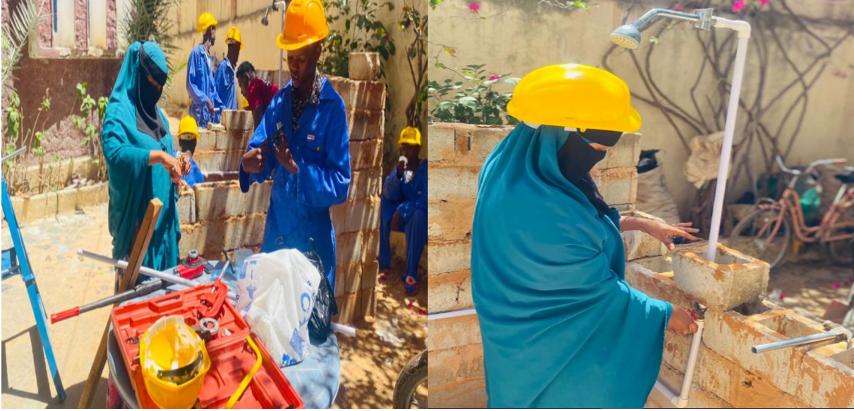
Plumbing and Pipe Fitting Practical Sessions
