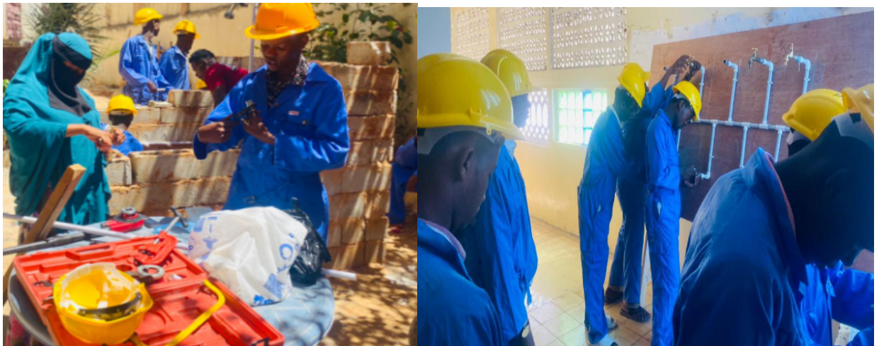
Plumbing and Pipe Fitting Practical Sessions
